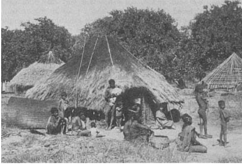
The Chenchu settlement of Pulajelma in 1940; during the dry winter season the round huts with conical roofs are being rethatched. In the background is the framework of a hut under construction.
