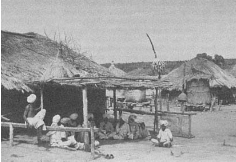
Gond village in the Adilabad highlands: the houses built of wood and bamboo are thatched with grass; free-standing cylindrical grain bins are made of wattle and covered with a mixture of mud and cow dung.
