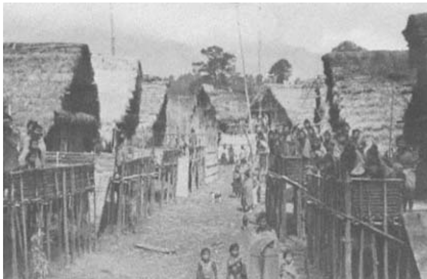
Street in a traditional Apa Tani village; the houses are built on piles and have verandahs in front and rear.
