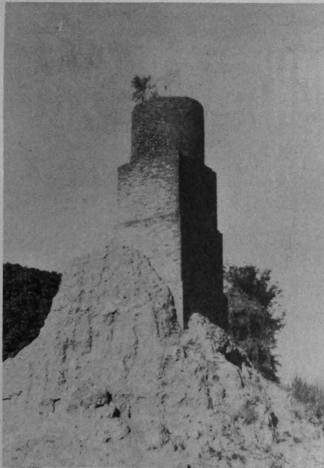
TITAORA, erected 1865, 16 m. north from Meerut, about \frac{1}{2} m. east of Muzaffarnagar road ; 30 ft. high, with isolated inner pillar. GTS. Trgn. 53 G ( 3 ) .
