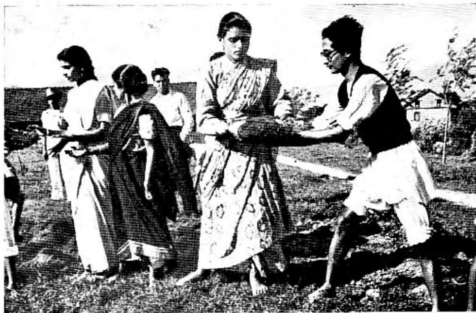
...building a footpath
