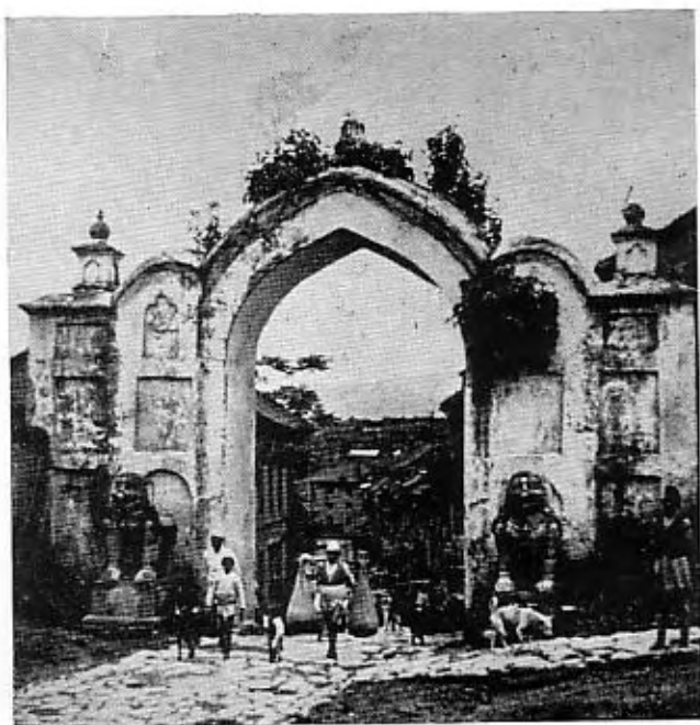
A typical entrance gate to a village
