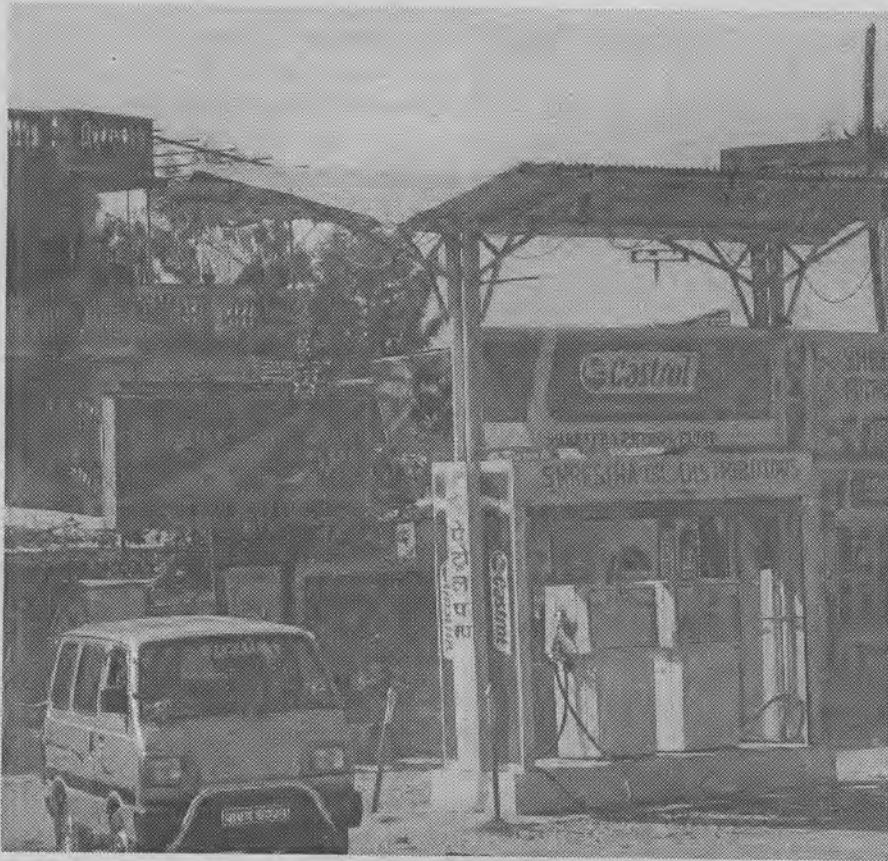
Petrol pump: No oil
