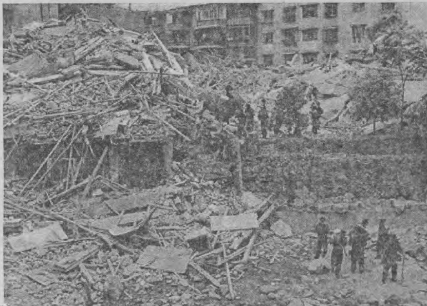
Collapsed buildings: Devastiated by quake
