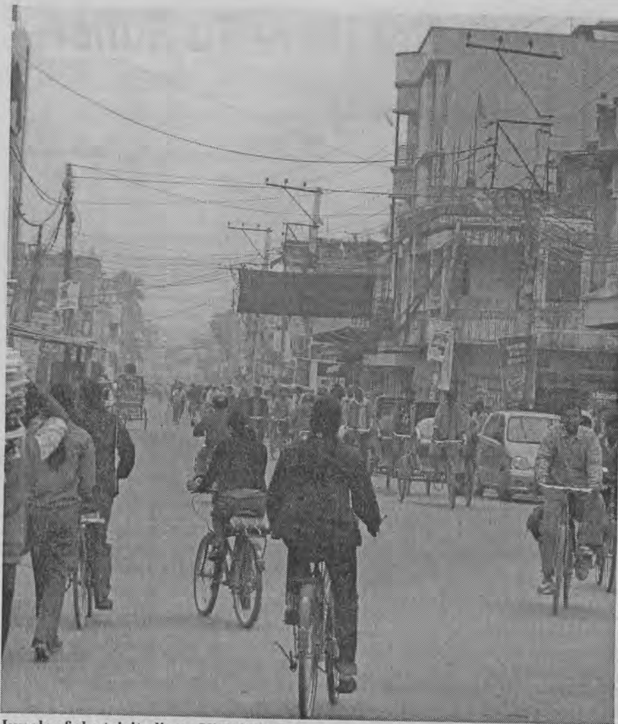
Jungle of electricity lines: High lackage
