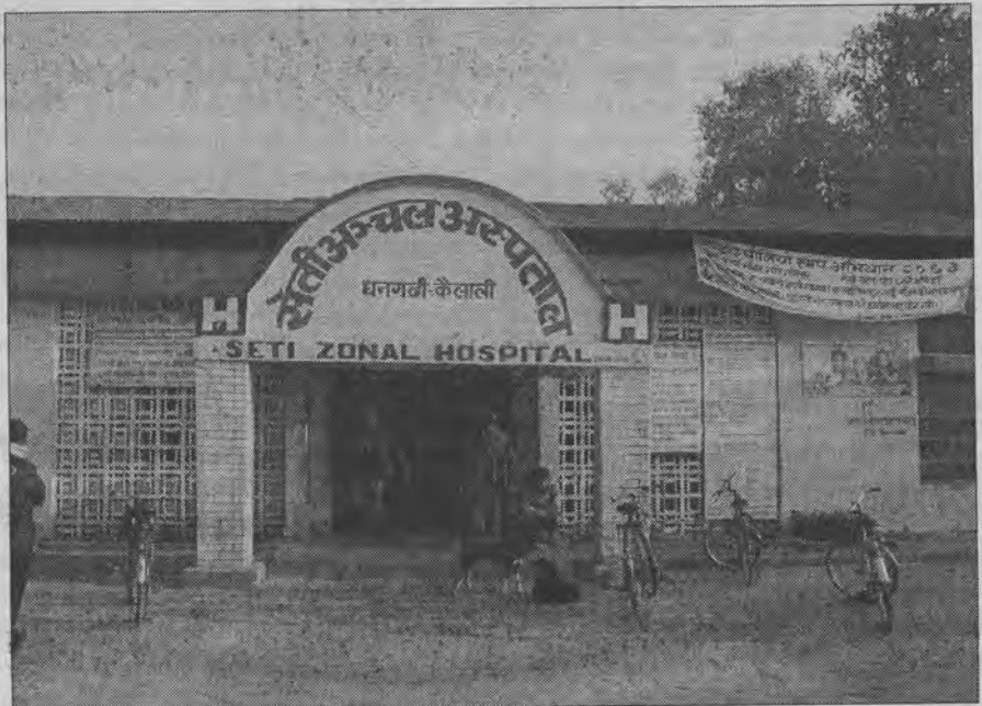
Zonal hospital: Inadequate manpower
