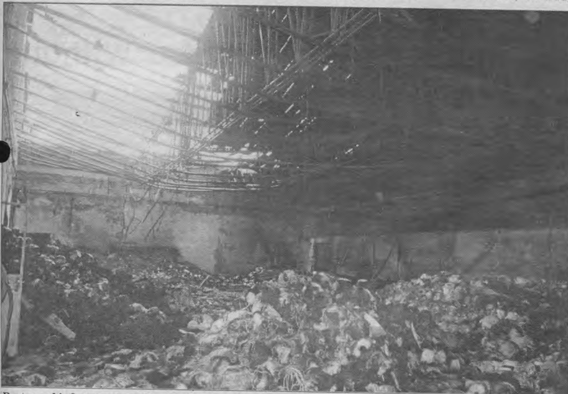
Destroyed infrastructure: Reconstruction effort imperative
