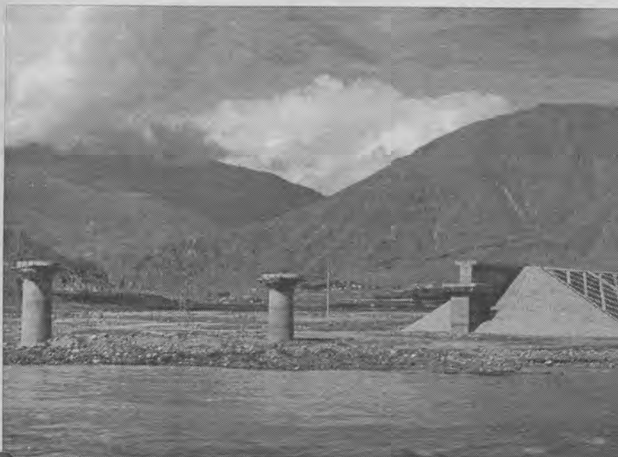
Railway bridge under construction: Miraculous technology Photos : Xinhua
