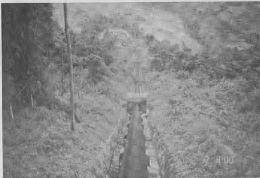
A drinking water pipeline: Rare infrastructure
