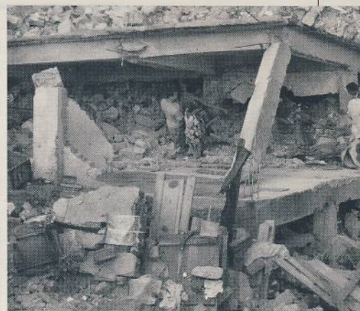
A demolished house
