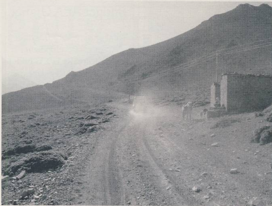
Road Under Construction
