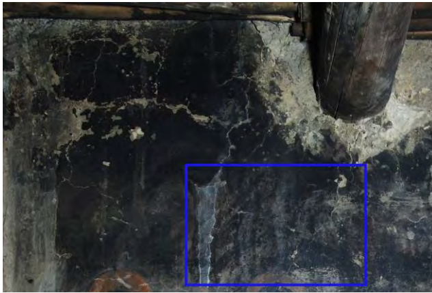
Fig. 7 — Detail of the south wall before cleaning; the blue square localize the next detail.
