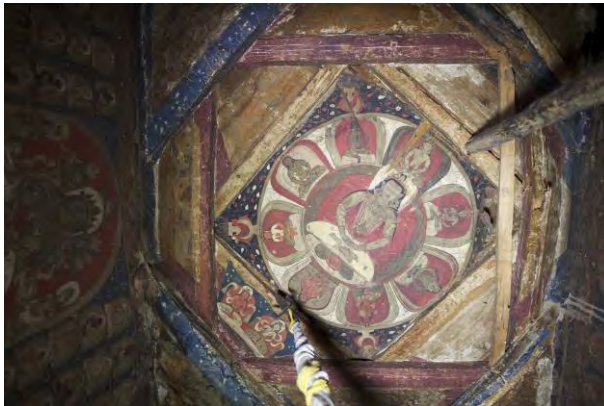
Fig. 10 — View into the upper chamber. (Bertsch 2012)
