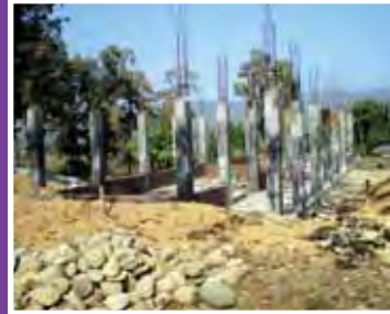
New building under construction
