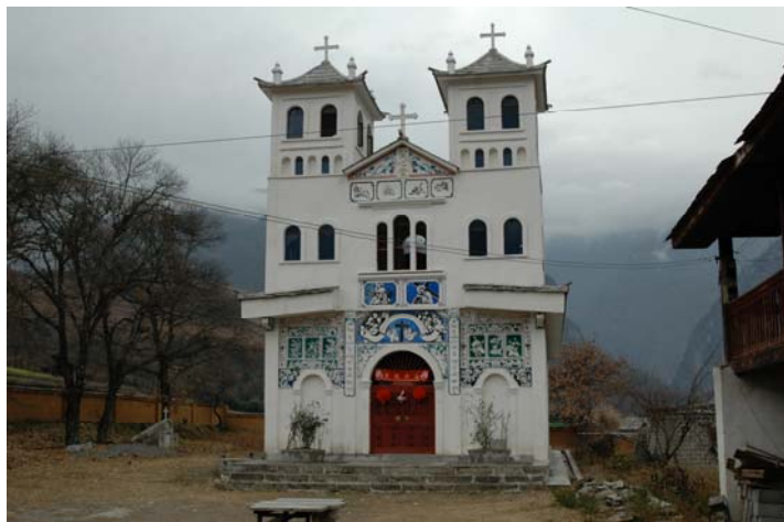
The Zhongding church in Bingzhongluo in Yunnan province.
