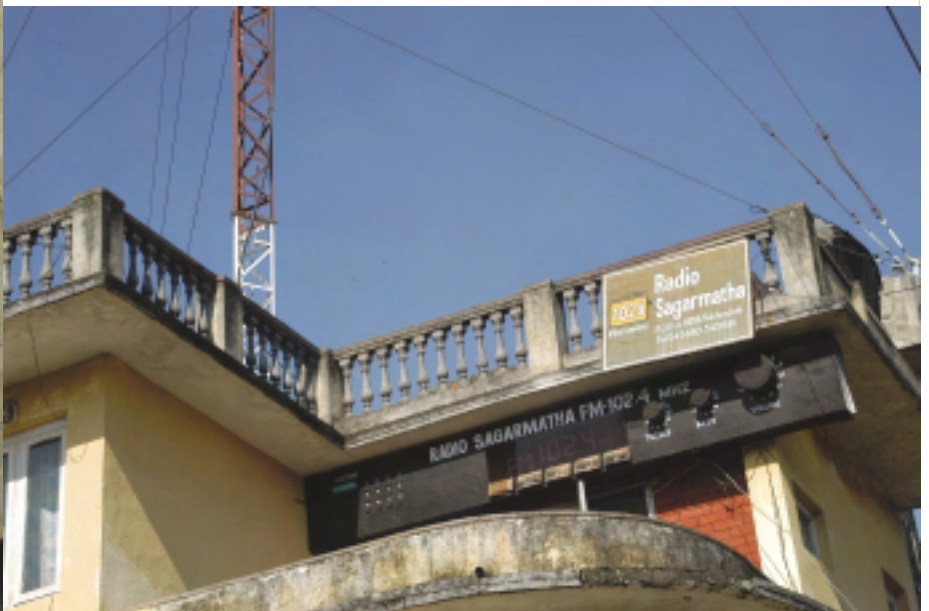
All photos: MW/SS
