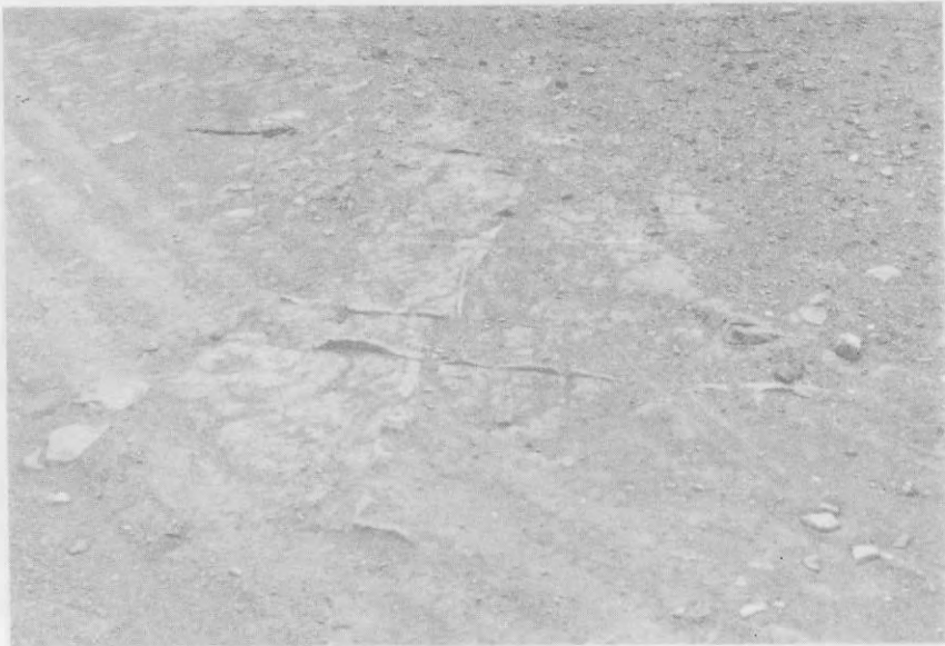
P-94 Shangs rDo-ring. Ancient foundations in the middle of the main road.
