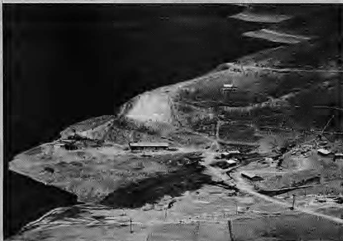
Construction site by the banks of the Yamdrok Yumtso.
