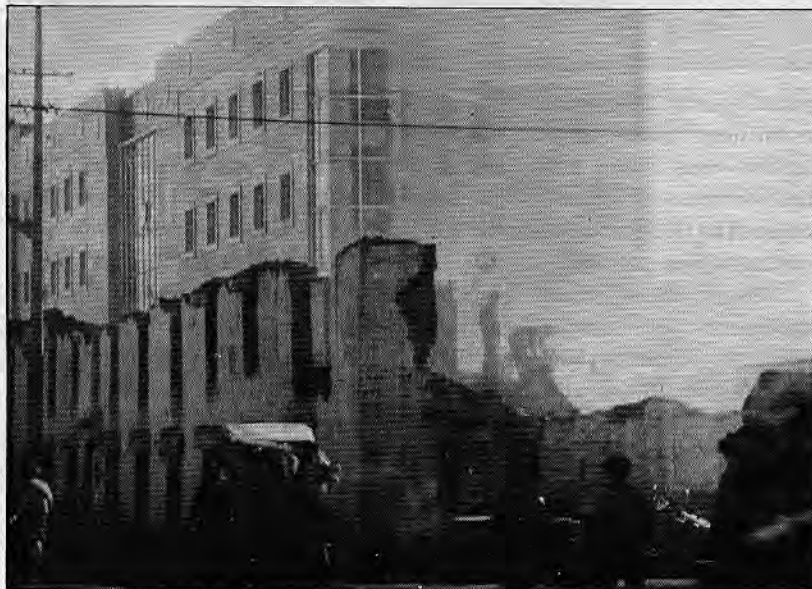
Demolition and reconstruction in Central Lhasa.
