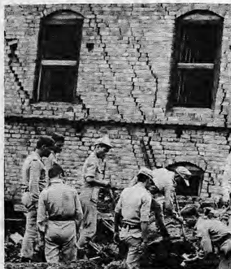
The 1988 Udaipur earthquake, (M=6.3) destroyed villages and towns in East Nepal such as Dharan, shown here.
