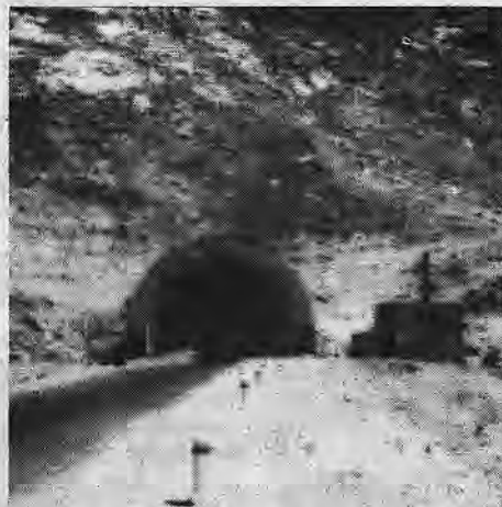
The north portal of the Salang Tunnel through the Hindu Kush. This tunnel, and an all-weather road, links Central Asia with South Asia. The 30-year impact of this road and tunnel has been greater communication between the two halves of Afghanistan, thereby reducing spatial inequalities among the many ethnic groups of the country.
