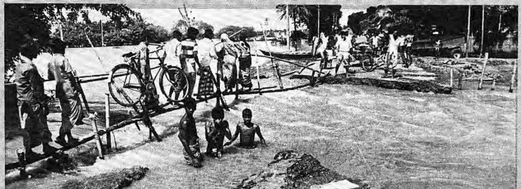
Flood-damaged road on Dhaka-Faridpur highway
