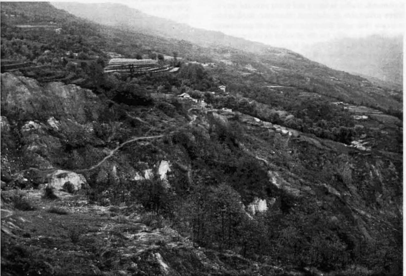
4 B. The landslide of Phalate, 12 years later (April 1994), has extended and is in the process of stabilization.
