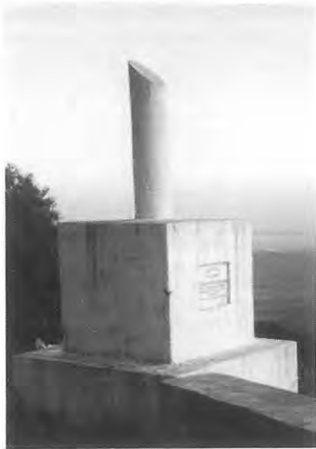
The Farrington tomb at Mussoorie demolished recently in a road-widening scheme
