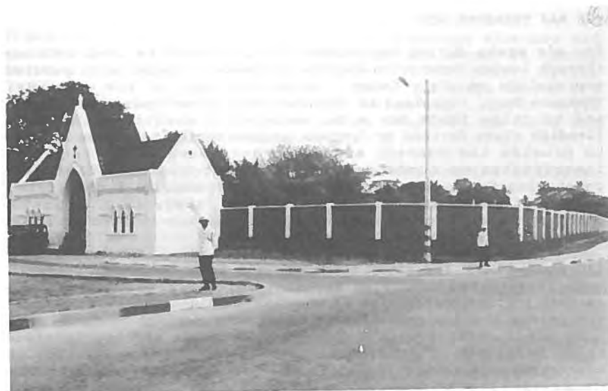
[Above] The newly restored gate-house and wall of the Cantonment Cemetery, Rangoon, Burma. BACSA provided funds for the work.
