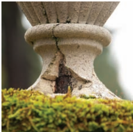
Grave of Hon Edward Gardner showing damage. © Dr Mark Watson.
