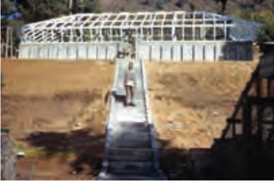
Glasshouse under construction at Godavari
