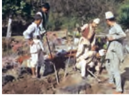
Rock Garden construction at Godavari
