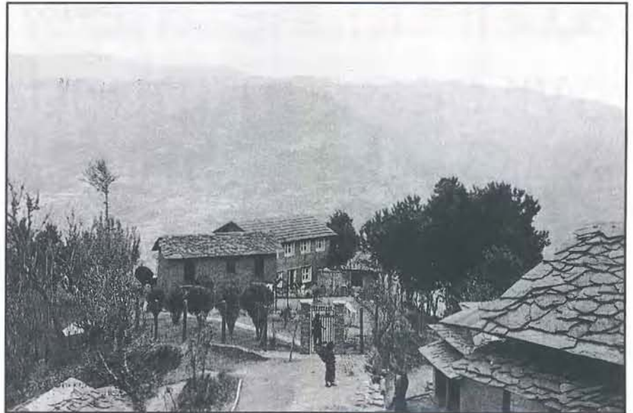
Remote Welfare Centre at Pirthi Set in the wilds of mid-eastern Nepal
