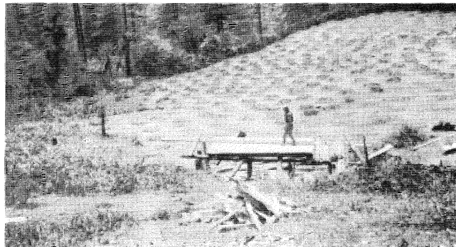
Plank sawing near Lamjura Pass
