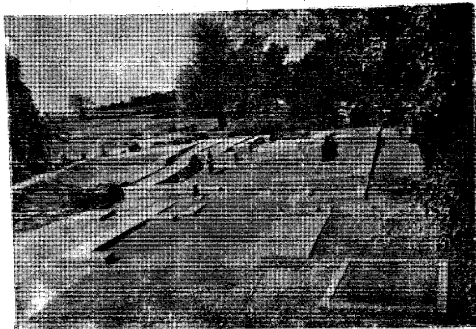
B. Western Gateway Complex After Conservation in V.S. 2034.
