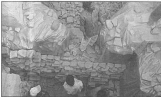
P.No.111a covering the trenches after completion
