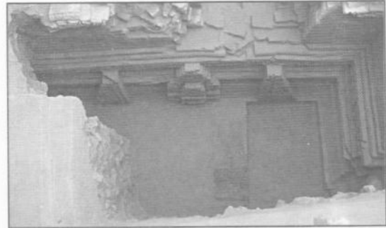
P.No.86 exterior projection of carved bricks of quadrant no. IV of G5 square
