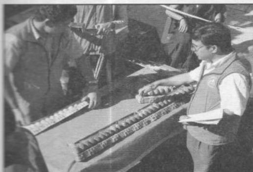
Listing, numbering and measuring removed copper sheets
