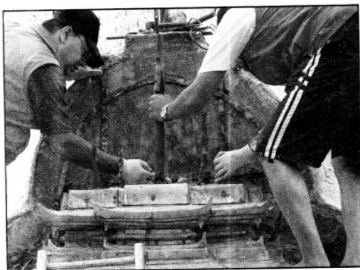
Workers are removing copper sheets for gold gilding
