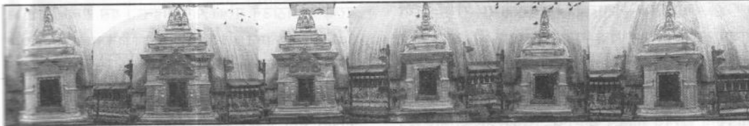
Niches shrines after conservation
