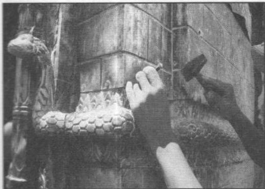
Using a hammer to take out the metal plates
