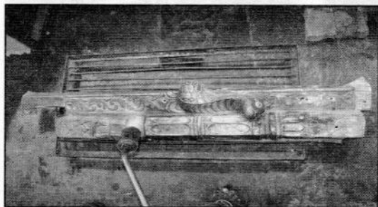
Heating one of the removed copper sheets
