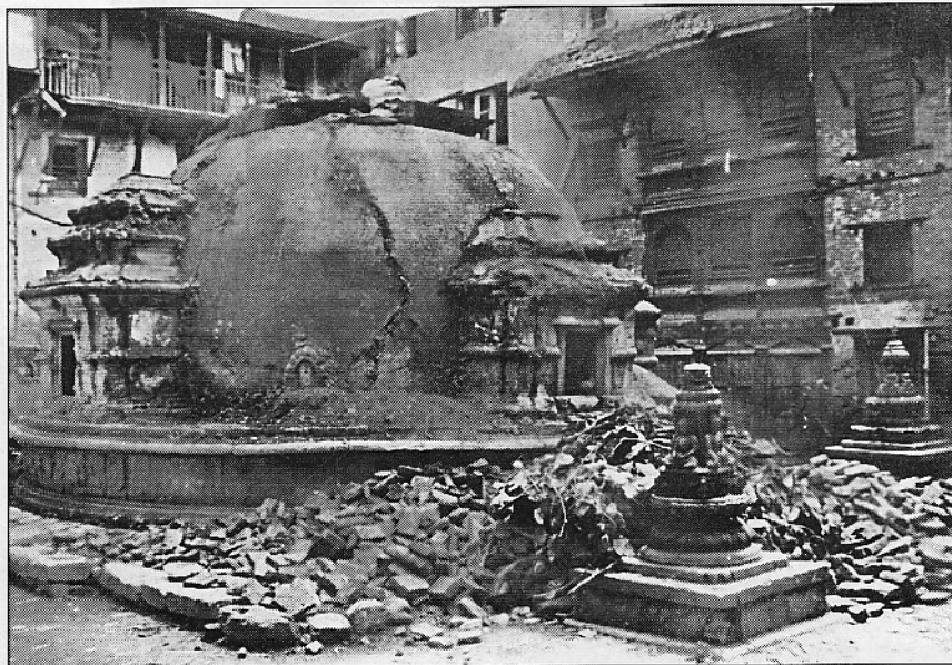
b. Stupa during renovation
