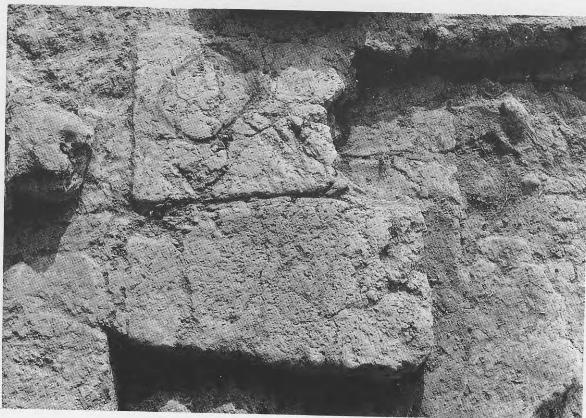
Fig. 12 - Gotihawa. Wedge-shaped Bricks of Stupa, One with Incised Circle.
