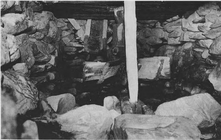
7. Thini watermill, showing chute, wheel and tenting rod
