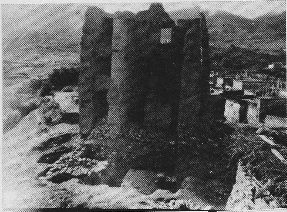
Ruins of DZARKOT Castle and Excavation Trench behind it.
