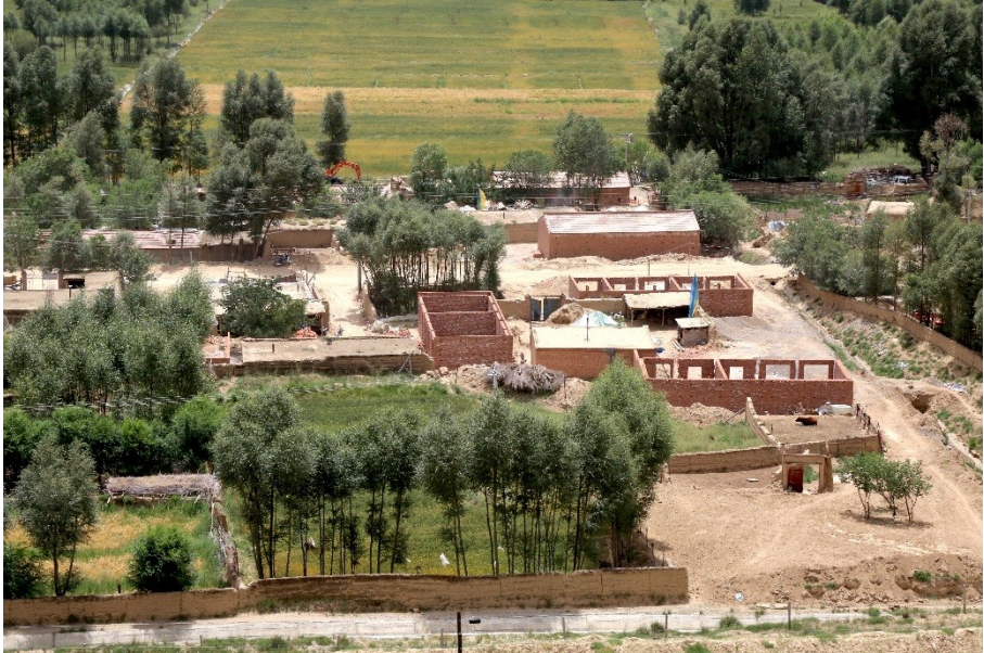
Photo 109. House construction in 2014.
