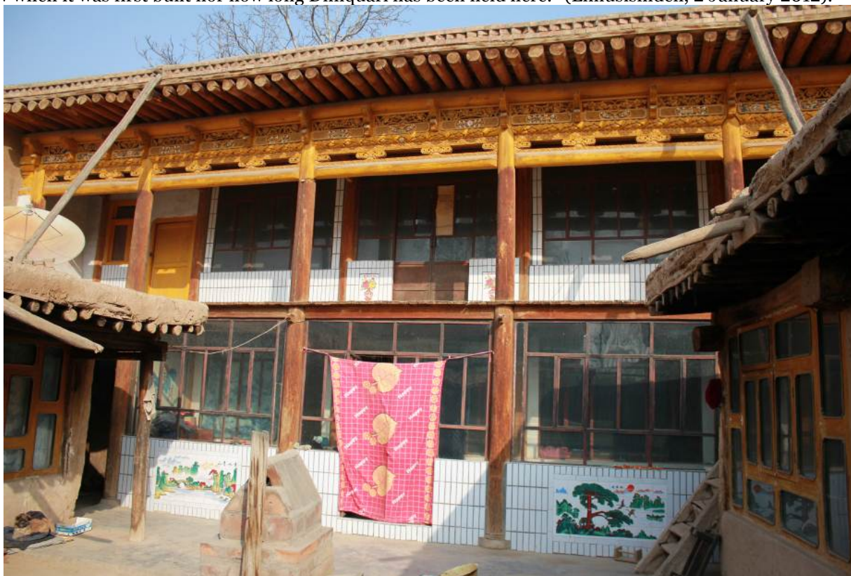
Figure 4. Huansuu's two-floor home. Diinquari is held on the second floor once every seven years. The home was renovated in 2005. Huansuu said, "Part of this building is several centuries old. None of my husband's relatives know when it was first built nor how long Diinquari has been held here." (Limusishiden, 2 January 2012).
