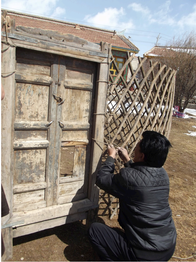
Figure 18. The door is joined to the last lattice panel, completing the frame.
