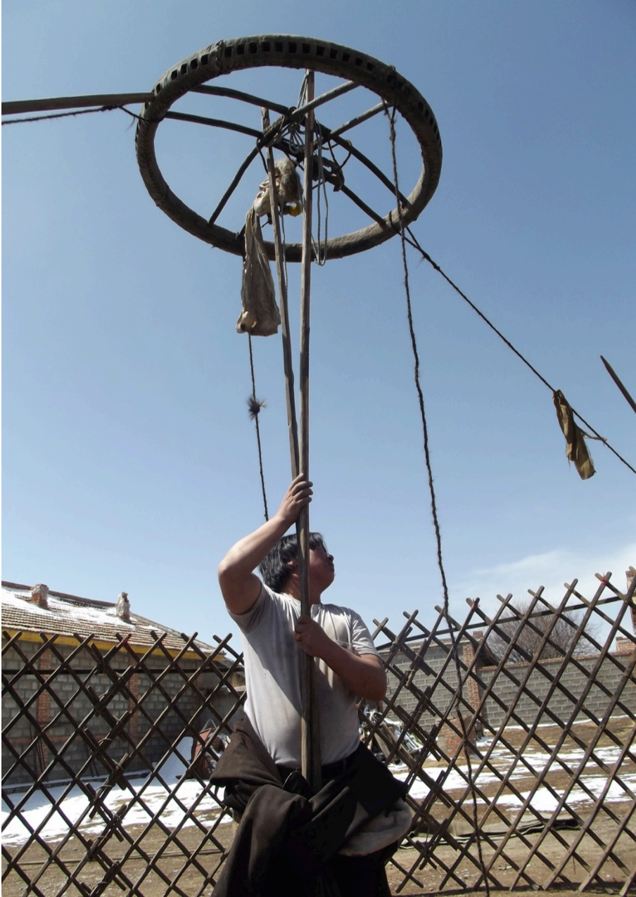
Figure 20. Raising the skylight.
