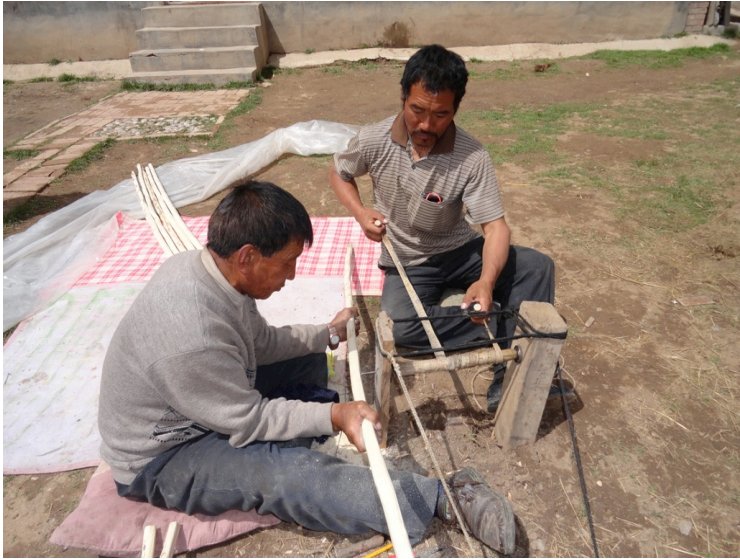
Figure 15. Two men operate the drill that makes holes in the poles.
