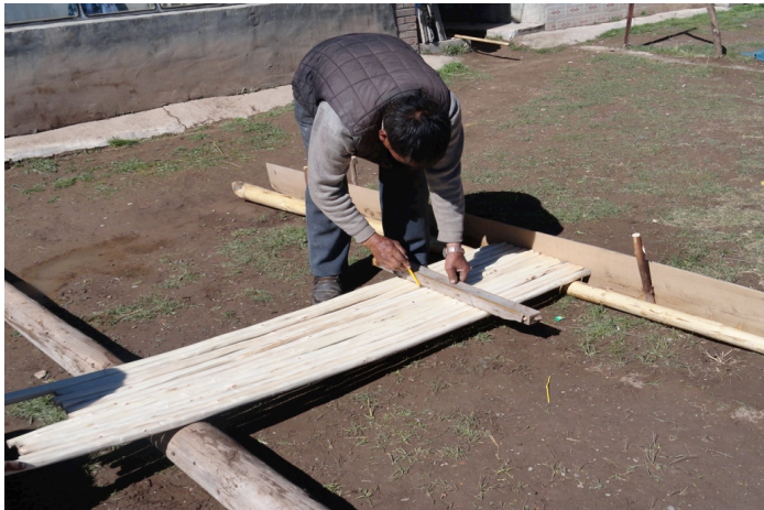
Figure 12. Measuring the poles to determine where holes will be drilled.
