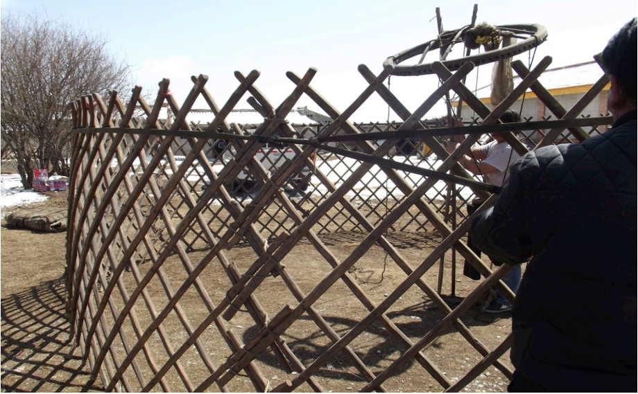
Figure 21. Binding the lattice panels together.
