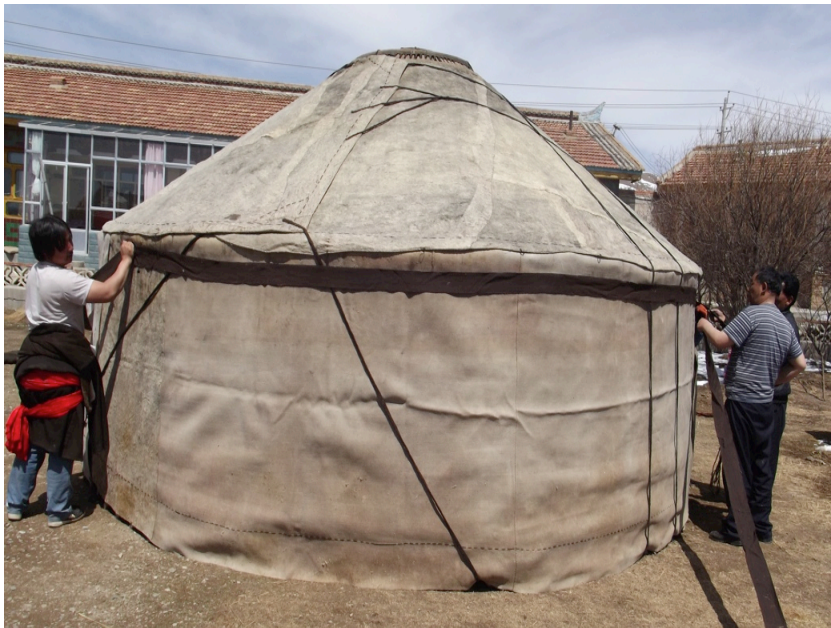
Figure 27. A 'belt' is tied clockwise around the yurt.
