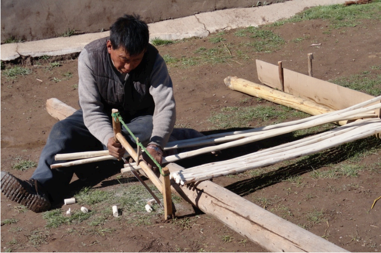
Figure 13. Sawing the poles to standard size.
