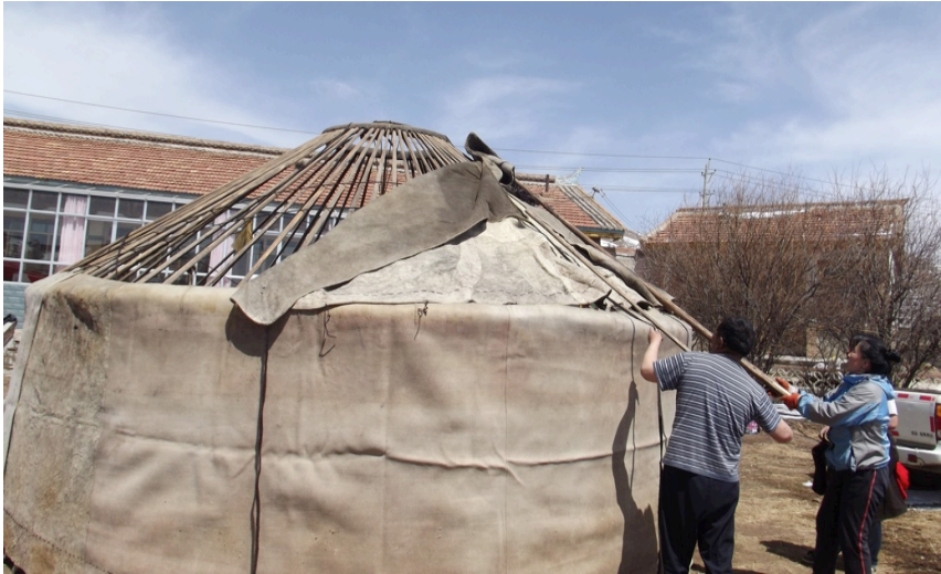
Figure 27. A 'belt' is tied clockwise around the yurt.
