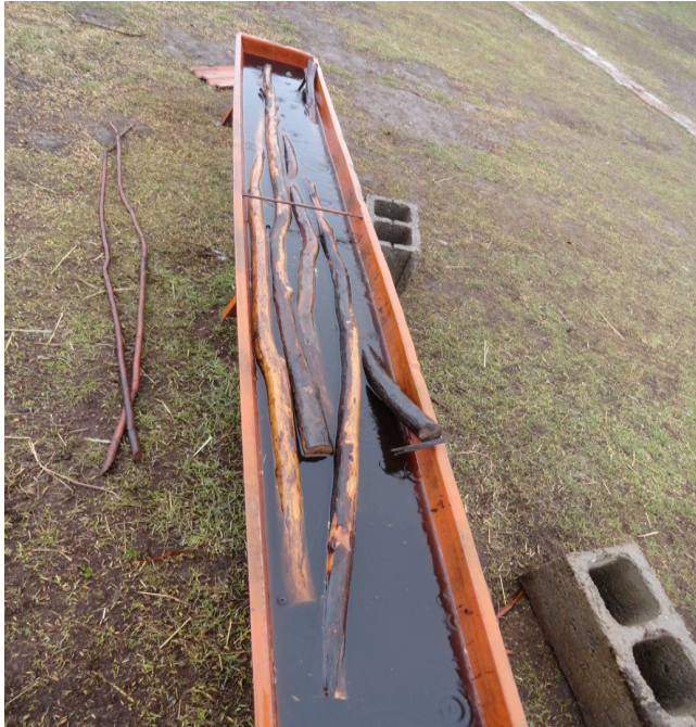
Figure 7. The willow branches are soaked in water to make them supple.
