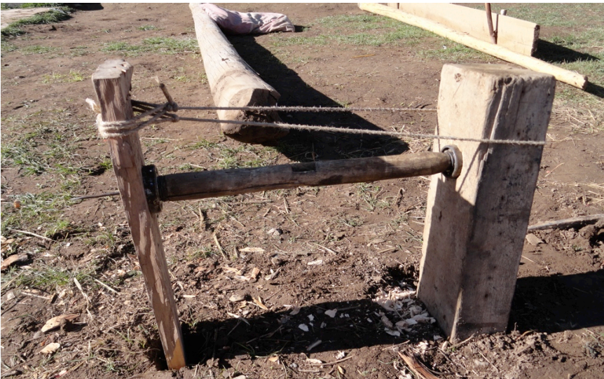
Figure 14. This ' bug ' drill is used to drill holes in the poles.
