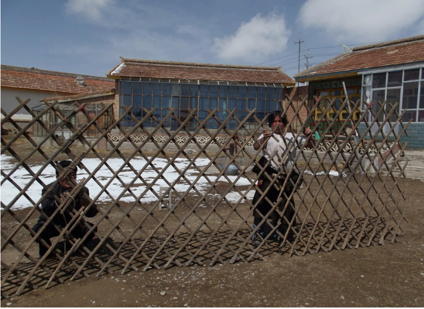
Figure 16. The man on the left uses a leather cord to tie the lattice pane. The person on the right puts a lattice panel in place.
