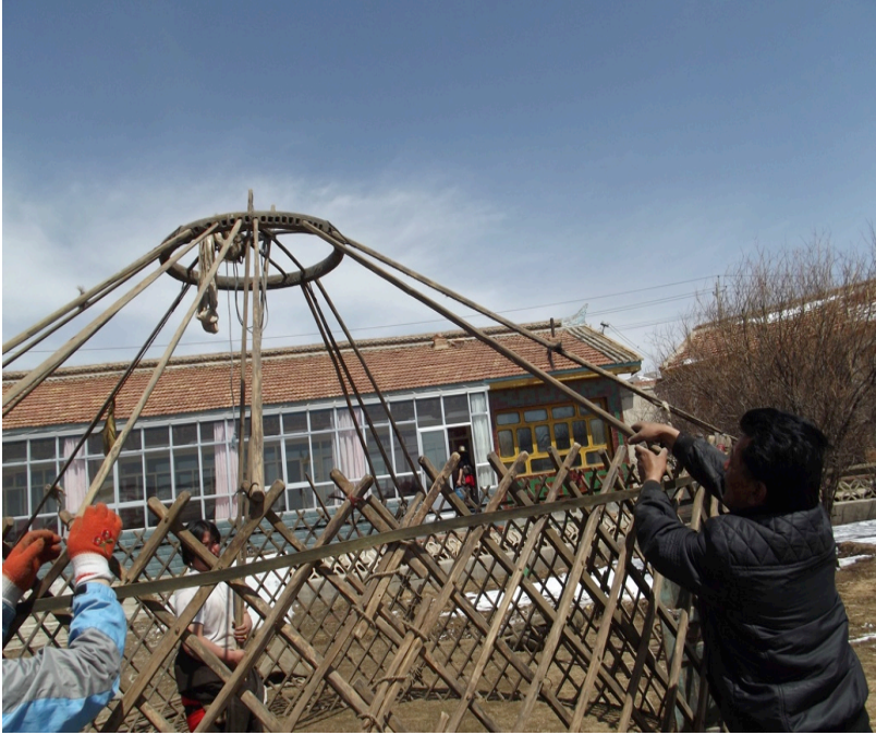
Figure 23. The yurt roof poles are inserted into the skylight in no set order.
