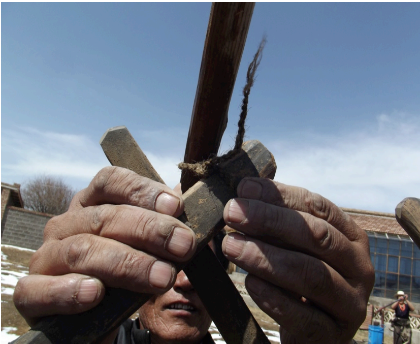
Figure 22. The roof poles are tied to the lattice panels with the left hand.
