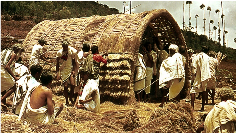
FIGURE 26. Re-thatching a dairy-temple at Inkitty hamlet, 1974. Photograph: Pauline Hetland Walker, ©The author.
