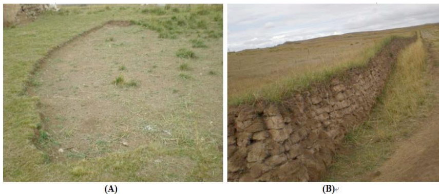
Figure 9. A grassland area used to produce sod bricks (A), and a sod brick wall/ fence (B).
