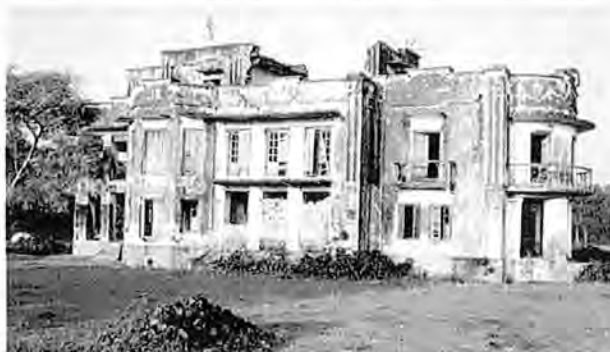
Fig. 40. Ruins of Banagai residence, W of Taulihawa, Kapilvastu. November 2006.
